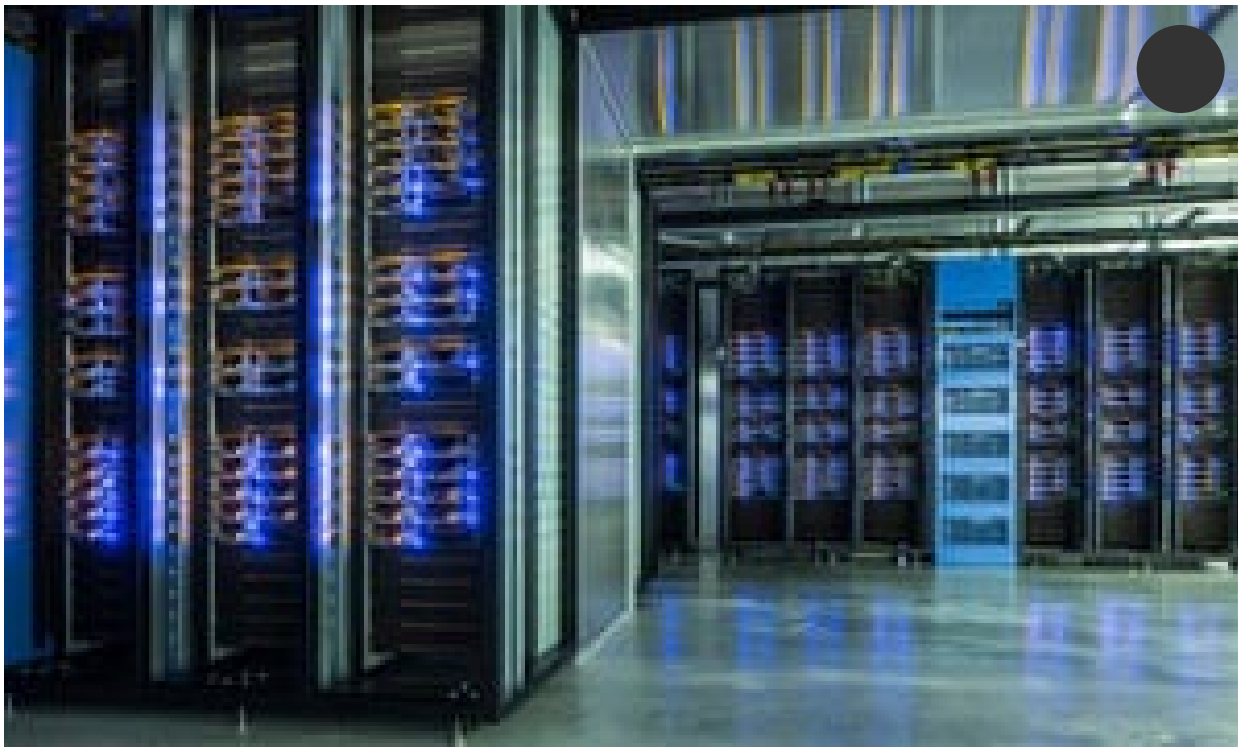
Facebook's Lulea data centre in Sweden, located on the edge of the Arctic circle, uses outside air for cooling rather than air conditioning and runs on hydroelectric power generated on the nearby Lule River. Photograph: David Levene/The Guardian
