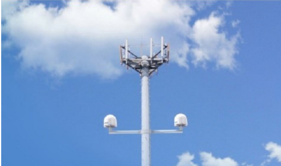
Picture 2: MNO tower-mounted OneWeb user terminals
