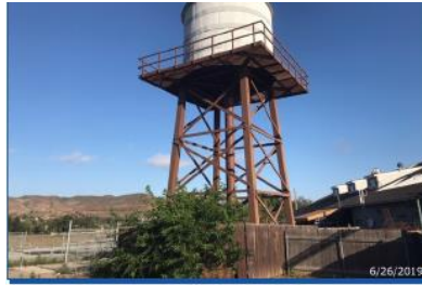
Photo 5 - Overview of existing faux water tank telecommunications facility, facing south.
