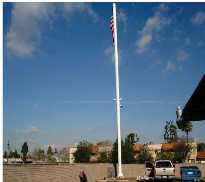
Figure 4 - Backhaul using 80' Flagpole Antennas
