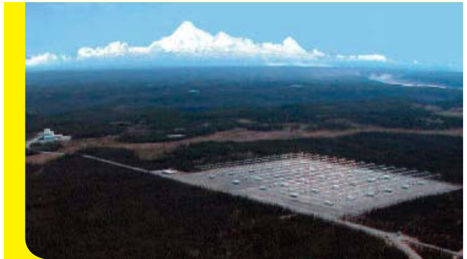
Fig. 25: HAARP location and construction.
